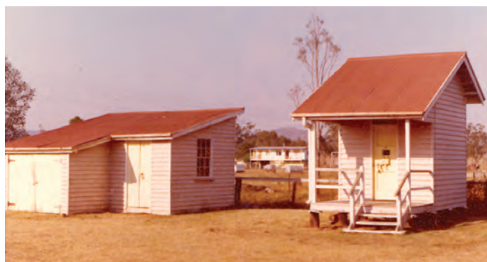
Nebo station lockup and garage 1979.
